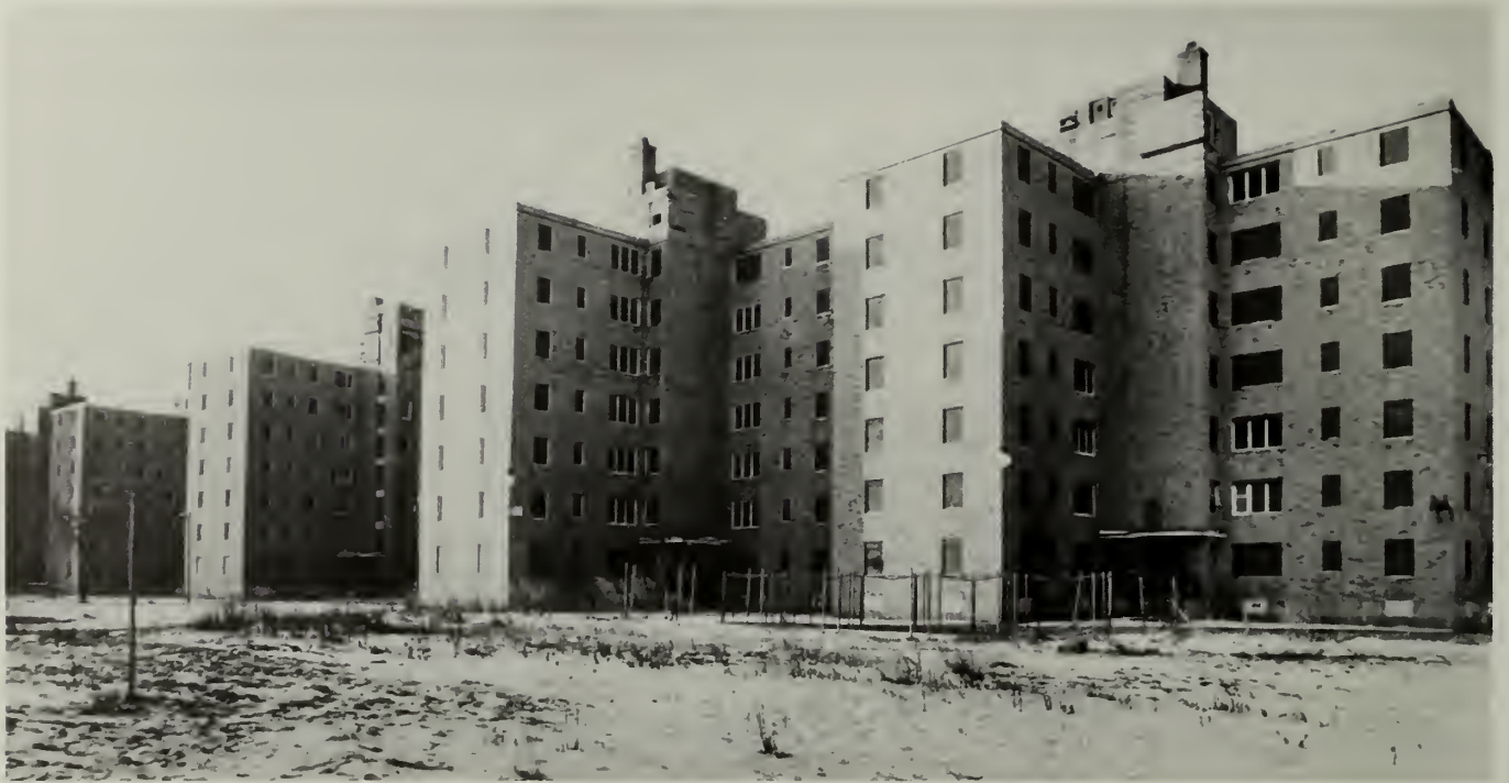
“Boarded-up high-rise building at Columbia Point stands vacant, the victim of vandalism and poor maintenance,” 1978. Boston Herald .
